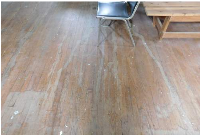
Figure 28 Detail of typical oak flooring condition.
