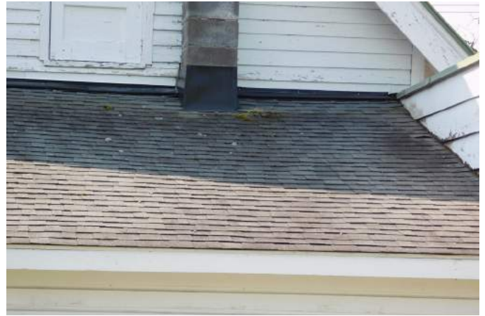
Figure 25 Asphalt shingle roof on addition.
