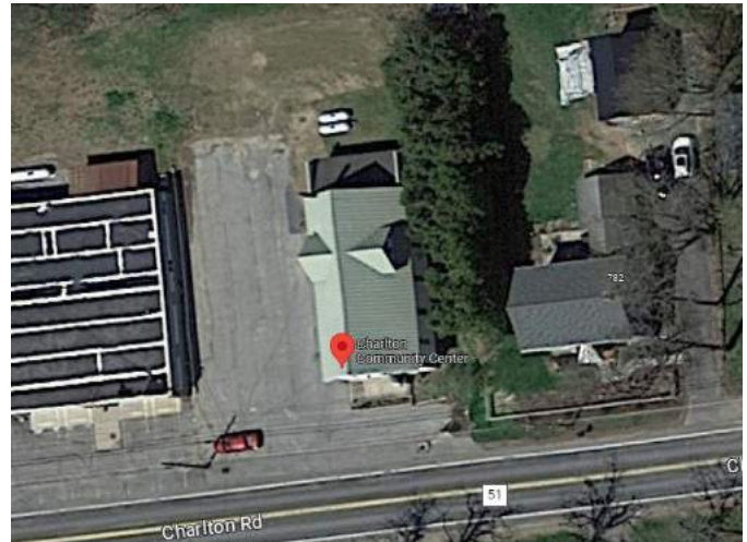
Figure 3 Aerial view of the site.
