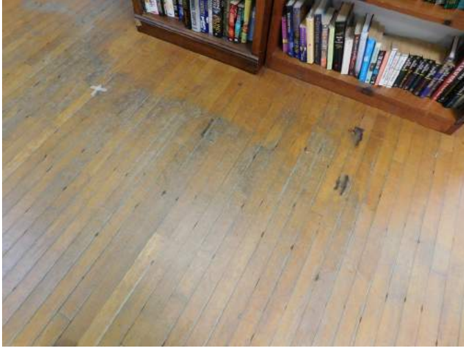
Figure 27 Detail of typical maple flooring condition.
