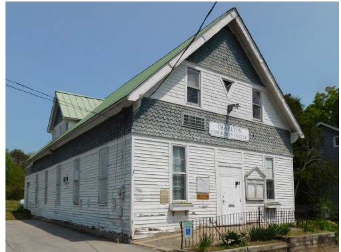
Figure 2 Current view of the south elevation of the Center.
