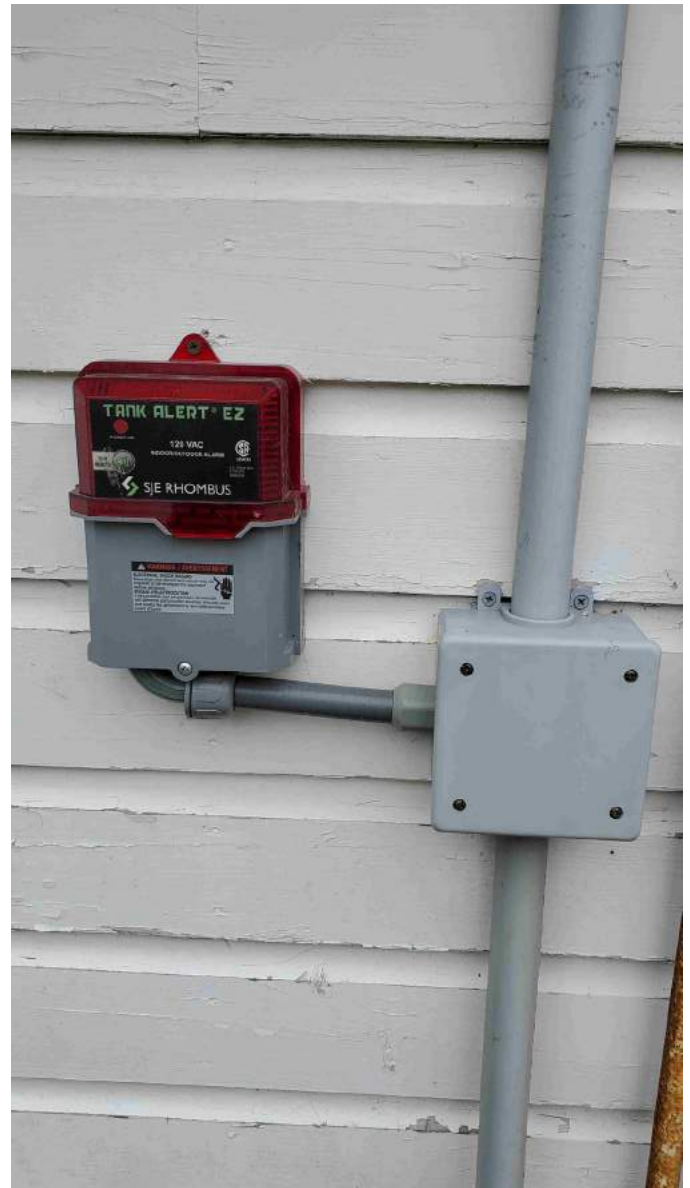
Figure 61 Raised Bed Pump Power
