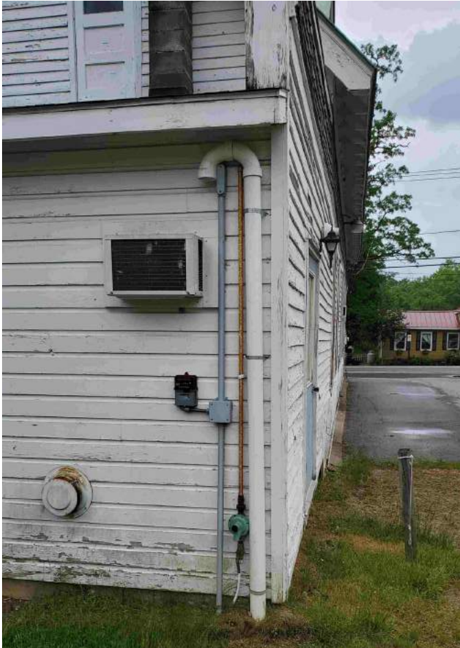
Figure 60 Raised Bed Vent
